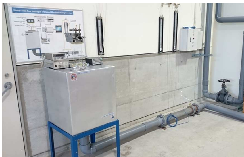
Fig. 28 Appearance of steady state flow test rig
